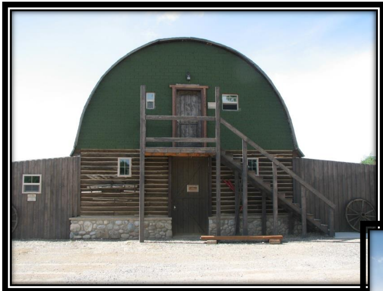
Back Entrance to the Barn
